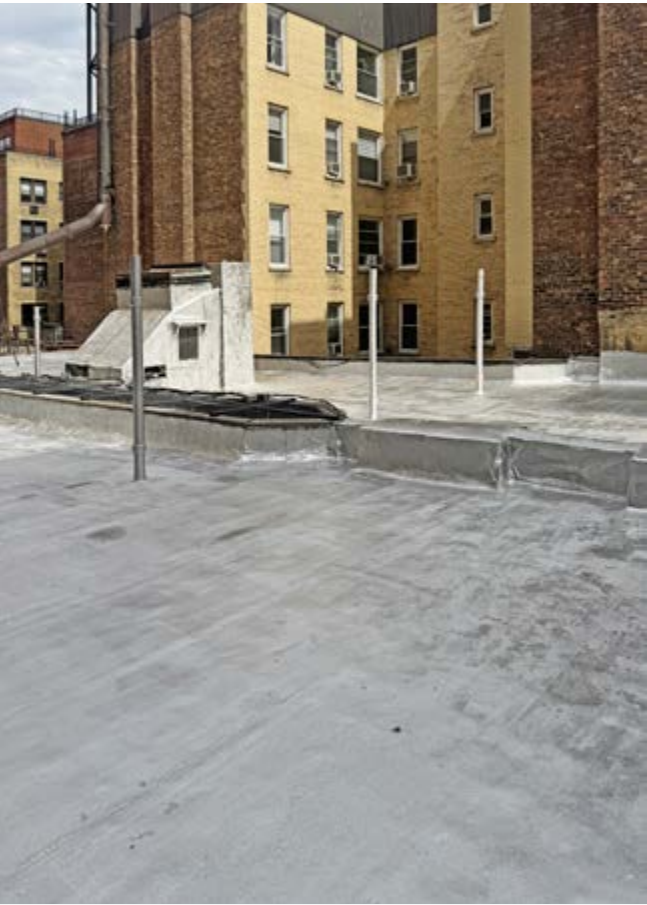
Exterior / Roof View
