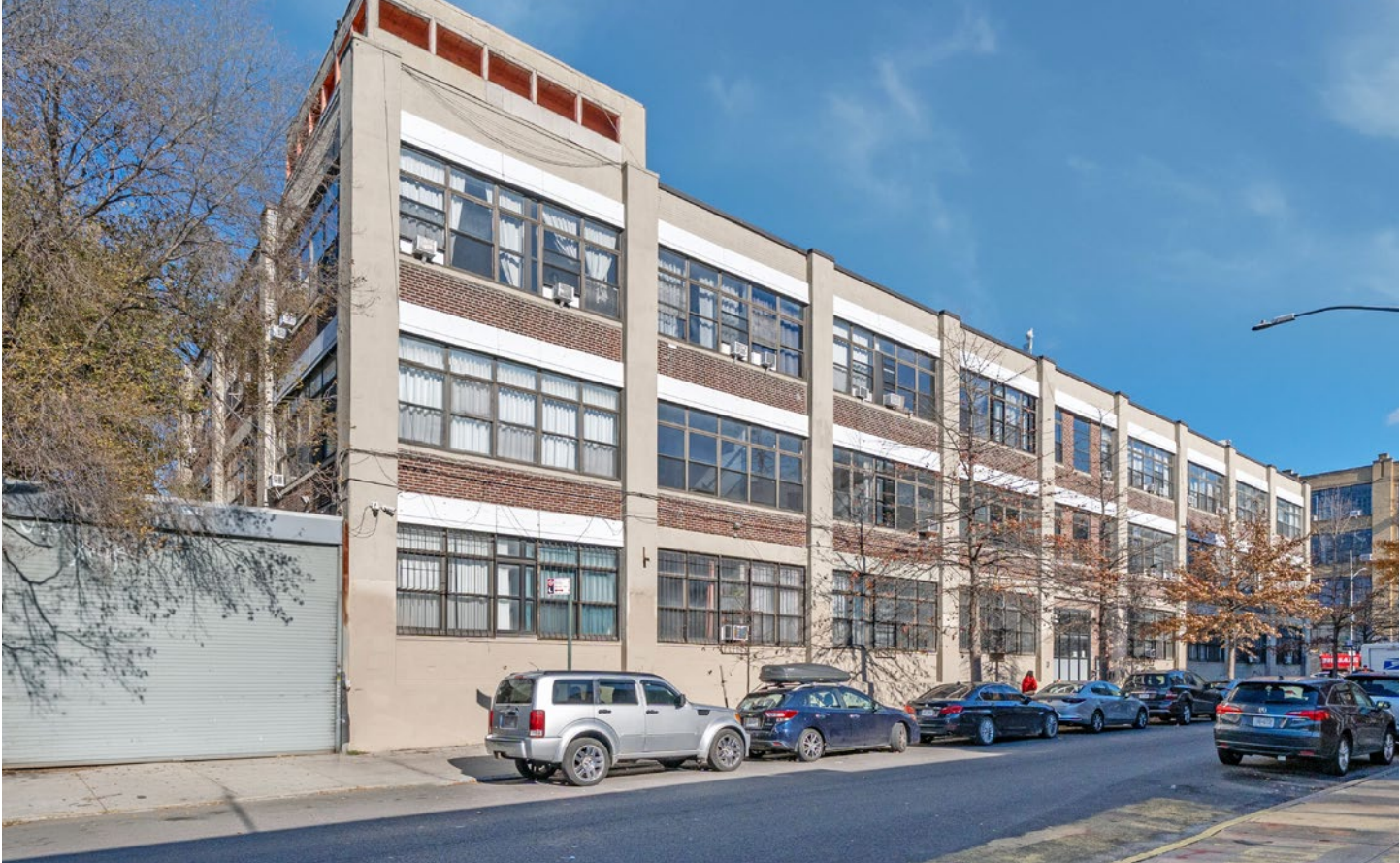
View from Seigel Street
