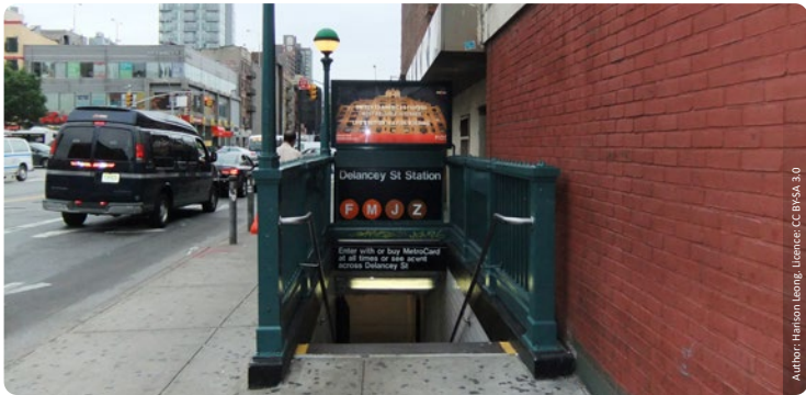
The entrance to Delancey Street station — F M J Z
